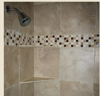
Shower wall tile with a 13”x13” tile laid straight with 4” linear accent of a cut down tile mosaic, as well as cut tile corner shelves
